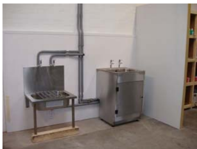
New sluice at Tottenham station
